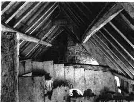
Boarding is not evident under each tie beam and is not historic in nature
