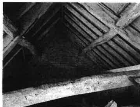
Boarding is not evident under each tie beam and is not historic in nature
